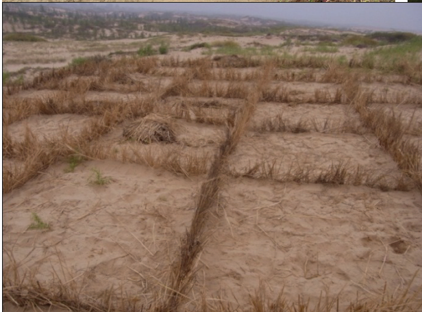
Fig. 4 Establishment of straw checkerboard barriers.
