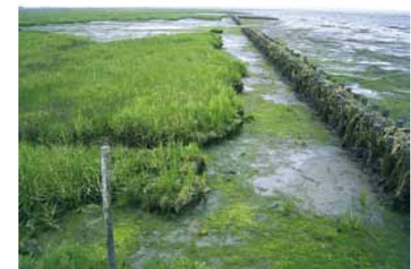
Figure 41: Land reclamation using fences on the German North Sea island Amrum (Photos: Albers)
