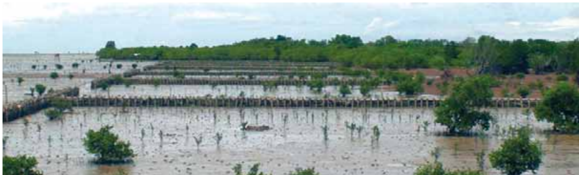
Figure 46: T-shaped bamboo fences on the coast of Bac Lieu Province (Photo: GIZ Bac Lieu)
