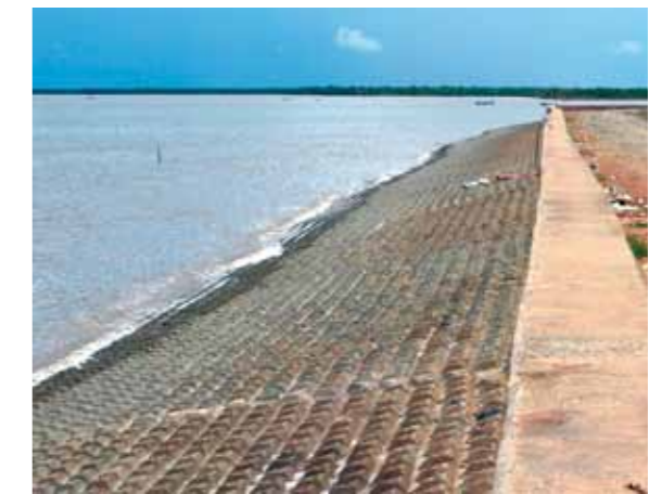
Figure 31: Steep slopes and rough surfaces of revetments hampers recreation activities at Ganh Hao, Bac Lieu Province (Photo: GIZ Bac Lieu)
