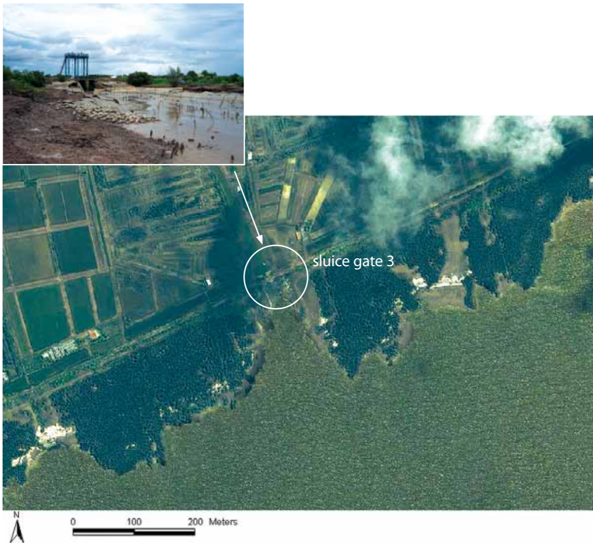
Figure 57: Funnel-shaped erosion at sluice gate 3 in Soc Trang Province (IKONOS Satellite Image 2012; Photo: Albers)
