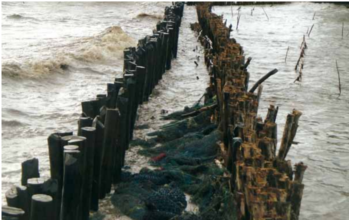
Figure 35: Wave breaking Melaleuca fence in Kien Giang Province (Russell et al., 2012; Photo: GIZ Kien Giang)
