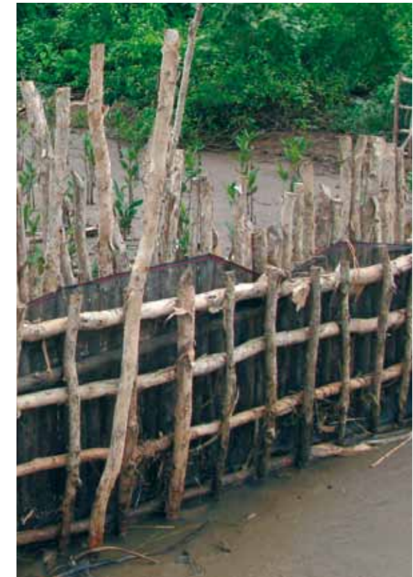
Figure 36: Sediment trap Melaleuca fence in Kien Giang Province (Russell et al., 2012; Photo: GIZ Kien Giang)
