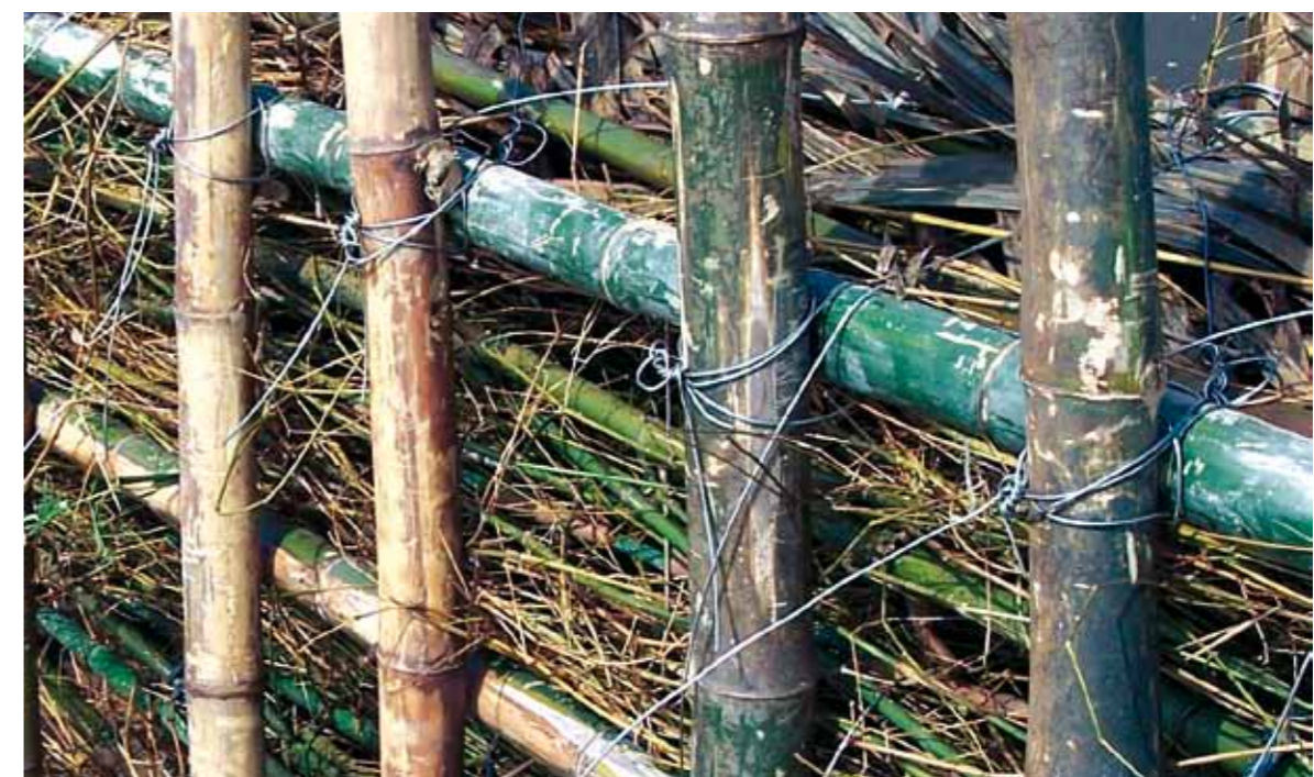
Figure 45: Joints made with stainless steel wire; (Photos: Albers)
