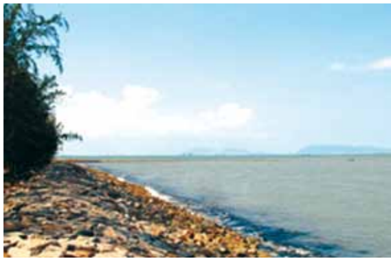
Figure 26: Revetment of natural stones on the coast of Can Gio District, Ho Chi Minh City (Photo: SIWRR)
