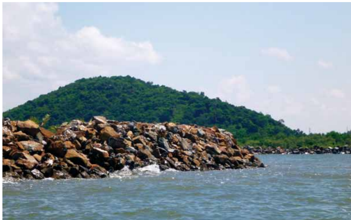
Figure 21: Detached rubble mound breakwater at Ha Tien in Kien Giang Province (Photo: Russell)
