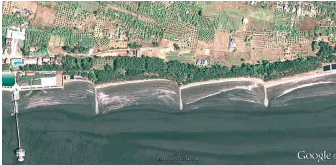
Figure 37: Rubble mound structure of an impermeable groin system at Can Gio District, Ho Chi Minh City (Satellite Image: Google Earth, Photo: SIWRR)
