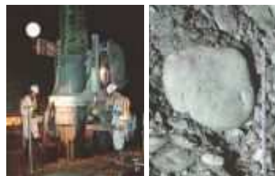
Press-in into Boulder Layer(D100 - 300 mm)
