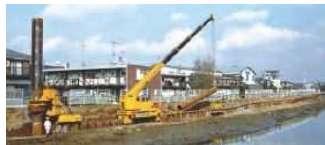
Build up Implant Structure Bank Protection with Kasetsu-less Construction
