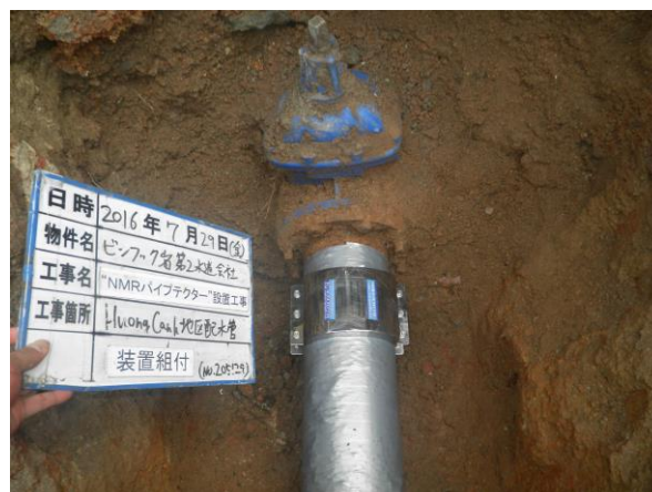
Water main supply pipe underground
