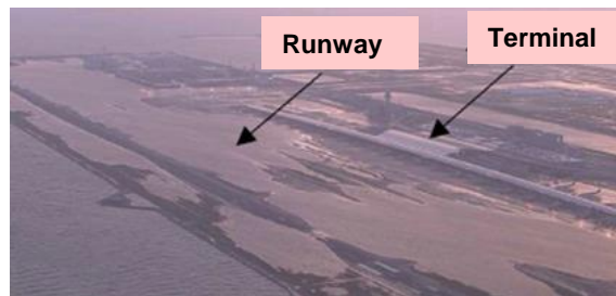
Flooded Kansai Airport Typhoon Jebi, 2018 (MLIT)
