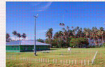
Equipment installed at Samoa meteorology headquarters
