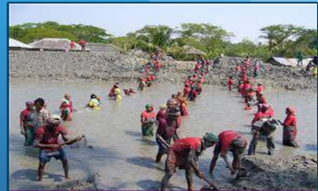
Rebuilding an embankment in Garbura (Photo by Ian Williams. December 07, 2009)
